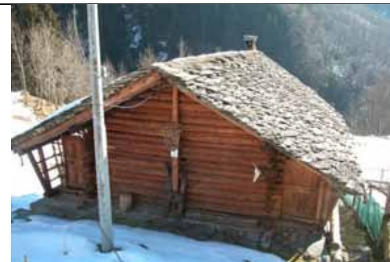
Baita a block-bau - fraz. Priami
