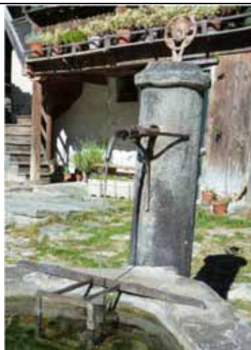
Pilastrino in serpentino proveniente da cave locali – Alagna, fraz. Pedemonte
